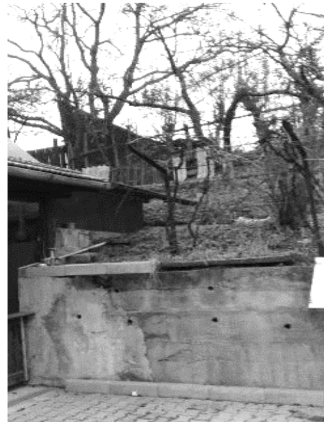
Figure 2. The second support wall.
