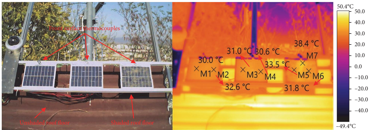
FIGURE 35: Thermal image showing front surface temperatures of the latitude-tilted PV test bed with some panels covered in dust on October 31, 2023.
