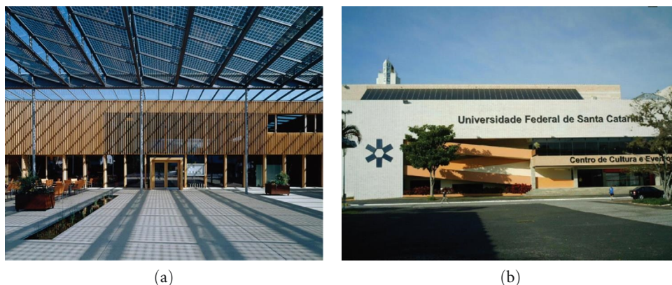
FIGURE 2: (a) BIPV providing a shaded area in Austria. Photo by Bruno Klomfar [22]. (b) BAPV at Universidade Federal de Santa Catarina in Brazil [23].
