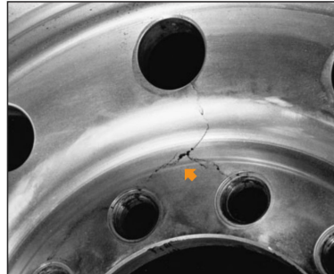
Figure 1. Crack growth near the rim hole illustrated by the position of the arrow.
