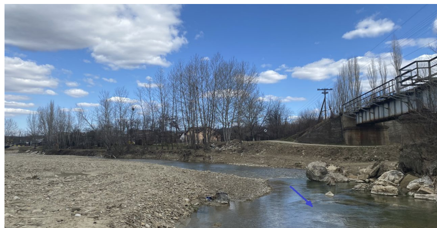
Figure 4. Bridge and the second embankment (150 m). The blue arrow indicates the flow direction.
