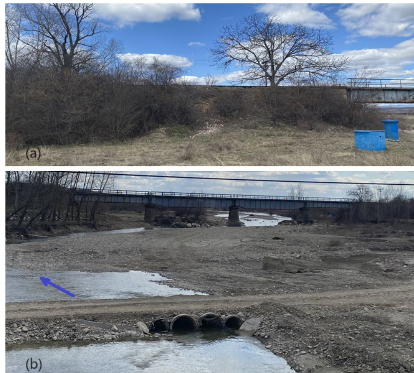
Figure 3. (a) Bridge over Vărbilău and the embankment; (b) bridge with three pillars and an opening of 100 m over the Vărbilău River. The blue arrow indicates the flow direction.
