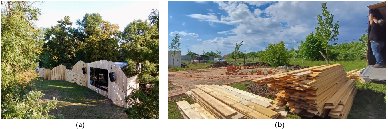
Figure 10. Material reuse—wooden plank recovered from the 2021 Plai Festival installation and reused in the Garden of Impermanence pavilion. (a) Temporary architecture at Plai Festival 2022; (b) Greenfeel site with recovered wooden planks from the wooden temporary installation at Plai Festival, 2022 edition. Image by arch. Amadeea Lazăr.
