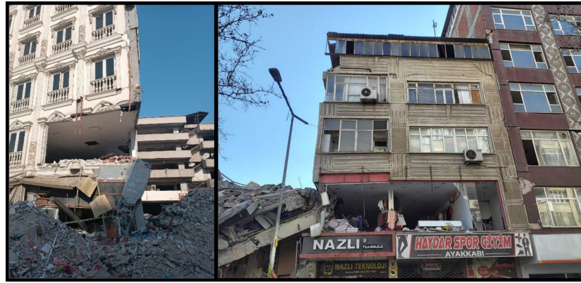
Figure 15. Damage due to the pounding effect.
