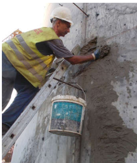
Figure 9. Removing wall defects with Penecrete waterproofing additive.
