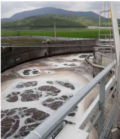
Figure 11. The wastewater treatment plant in-service.
