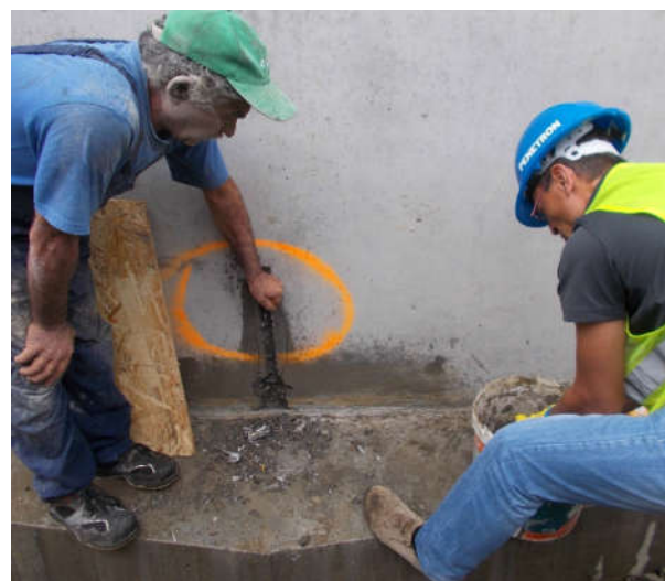
Figure 10. Removing wall defects with Peneplug waterproofing additive.
