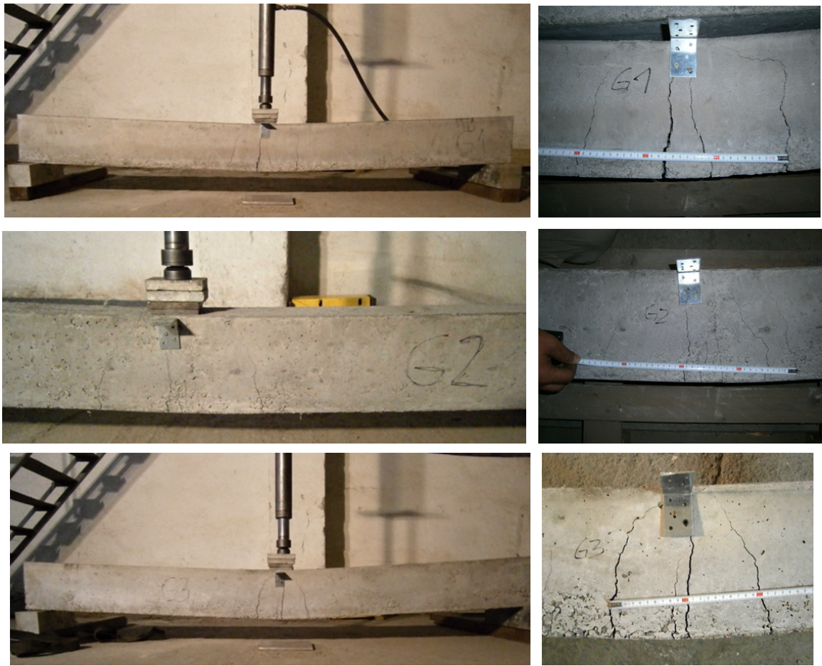
Fig. 3. G1, G2, G3 concrete beams and cracks
