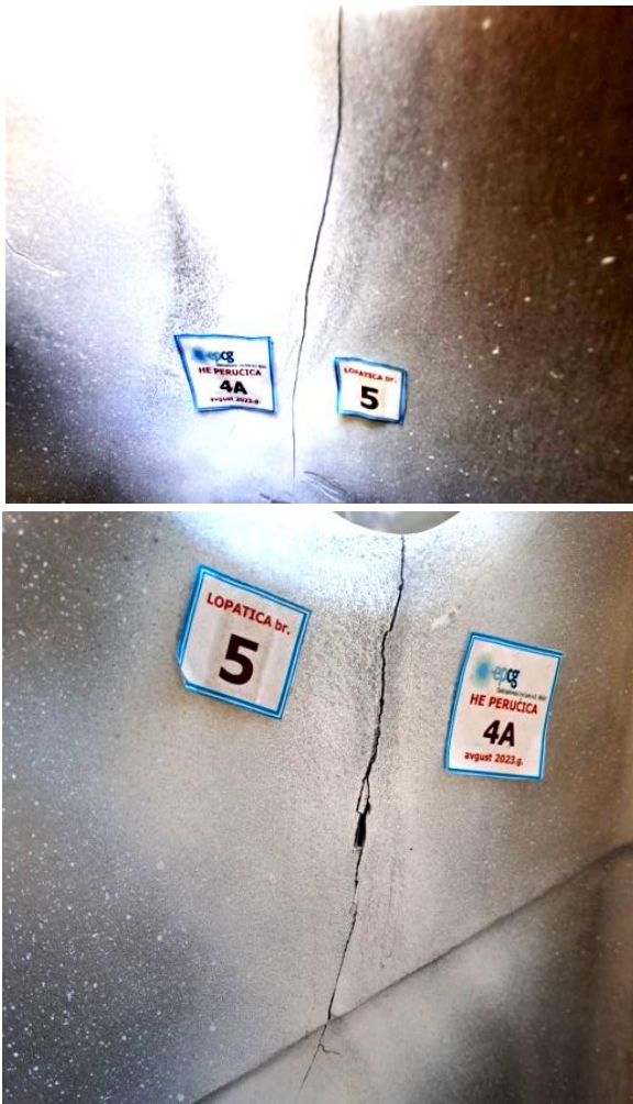
Figure 3. Detected crack on Pelton runner's blade, 200 mm length: front side (top); back side (bottom).
