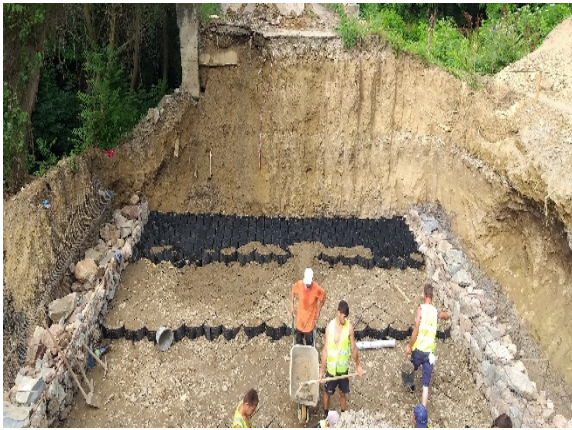
c. Geosynthetic sand gabions executions.
