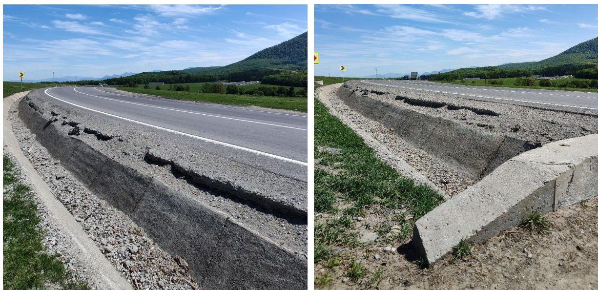
Figure 4. E68 (DN1)—curved road sector used for the study.
